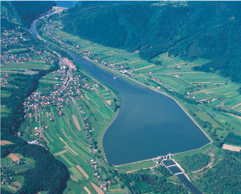
Fig. 1. Czaniecki Reservoir and Czaniec Dam
