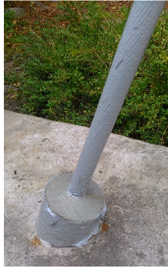
Fig. 3. Fastening rope in sleeve with thread Fig. 4. Anchoring guy in reinforced concrete block
